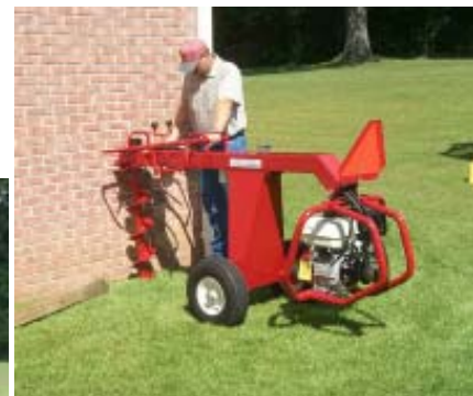
Figure 11B Up-close Drilling
