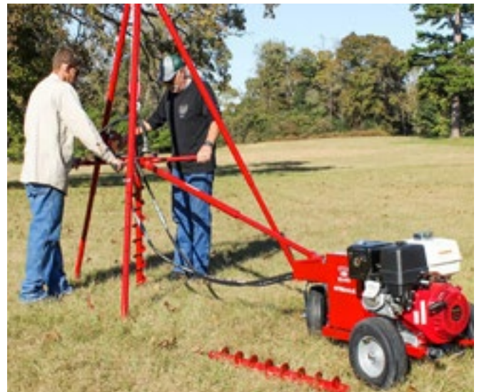
Hydraulic Earth Drill being used with a Lifting Frame
