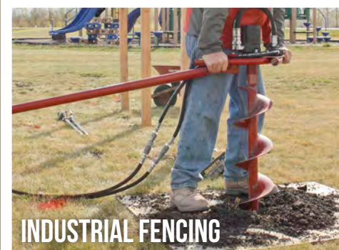
FOUNDATION PIER HOLES
